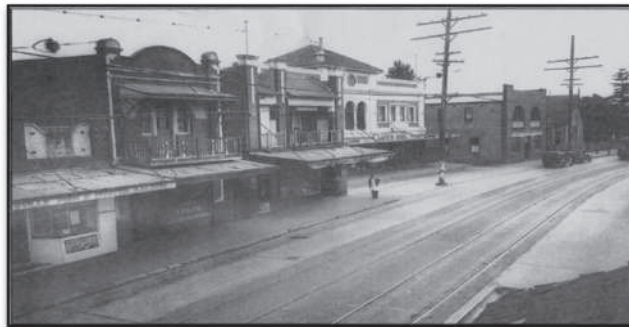
Figure 9. Looking north along Victoria Road c. 1939. (Source: National Library of Australia, http://trove.nla.gov.au/work/191374185?q=gladesville+hotel&c=picture&versionId=208854388 , accessed 13 August 2015).
