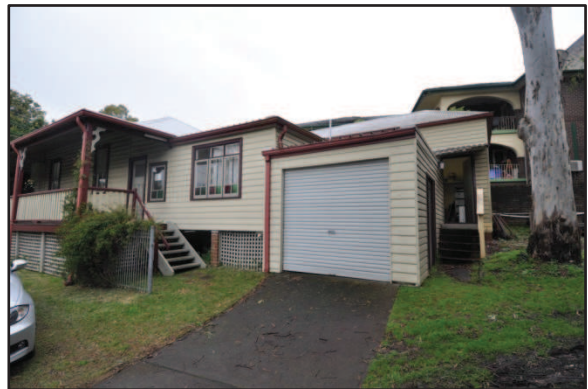
Figure 24. View of the Flagstaff Street elevation of the cottage at 10 Cowell Street, showing the rear extensions including the garage. (Source: Heritage21, July 2012).
