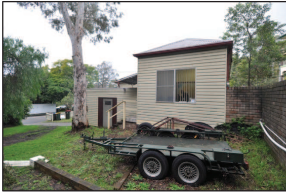
Figure 25. View of the rear extensions to the original timber cottage at 10 Cowell Street, looking south. (Source: Heritage21, July 2012).
