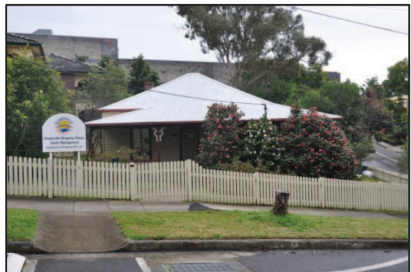
Figure 22. View of the building at 10 Cowell Street, which has been recommended for local heritage listing. The photograph shows the Cowell Street elevation. (Source: Heritage21, July 2012).
